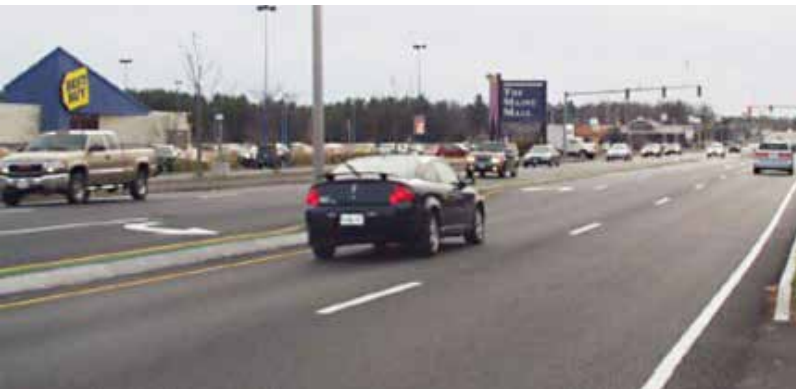
Part of Maine Mall Road was repaved with pervious pavement, part of a broader set of green infrastructure projects that are helping to restore Long Creek.
